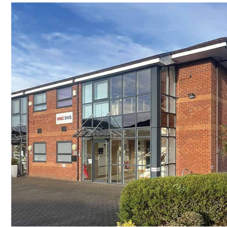
KWC DVS Northern Office, Chesterfield, UK
