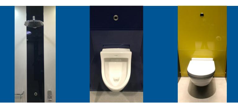
The programmable sensors on site can be fully customised to suit using the Handheld Programmer, allowing for different settings to be applied to products to best suit the stadiums needs. We now have urinals with the shortest possible "walk away time" ensuring a full flush as often as is required to clear the bowl. The flush has also been optimised to save water whilst not compromising performance.
