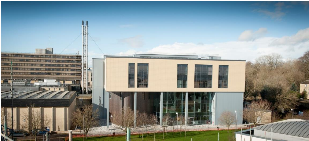
The Chancellor's Building, University of Bath
